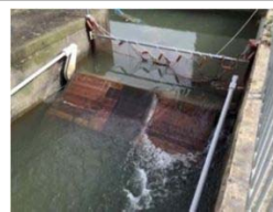
剥離流抑止板＋寒冷紗 ⇒底生魚遡上促進
