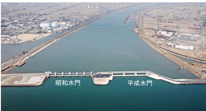
昭和 water gate と平成 water gate
