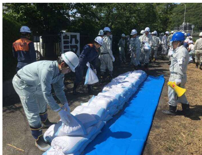
[改良積み土のう工]
