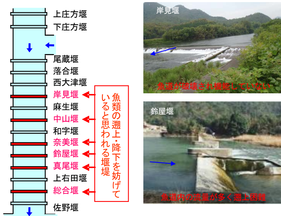
図3.2.3 魚類等の遡上・降下を妨げる堰堤
