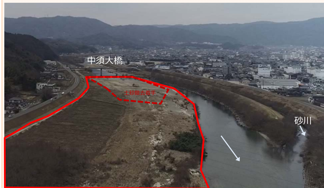
樹木伐採状況 (H31.2)
