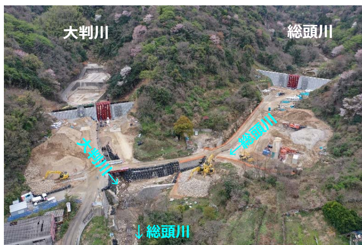
総頭川・大判川施工状況 (R2.3末時点)
