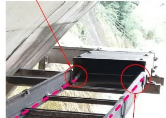
Optical Fiber Cable Cut Situation (Starting Point)
