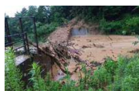
▲井口台4号砂防堰堤
