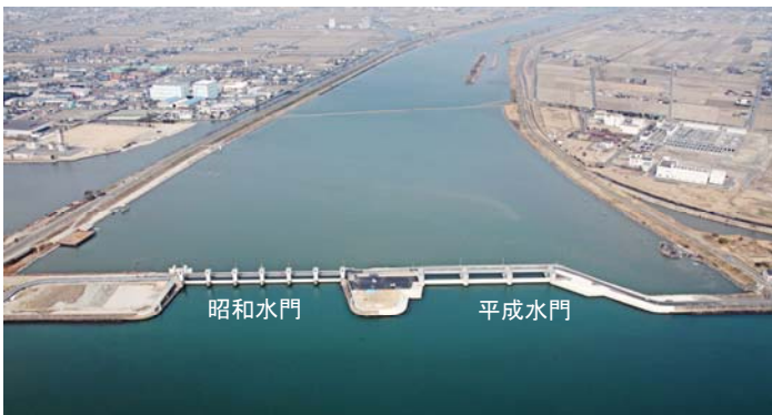
昭和 water gate と平成 water gate
