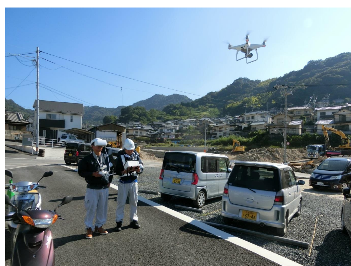
Investigation of disaster situation by drone
