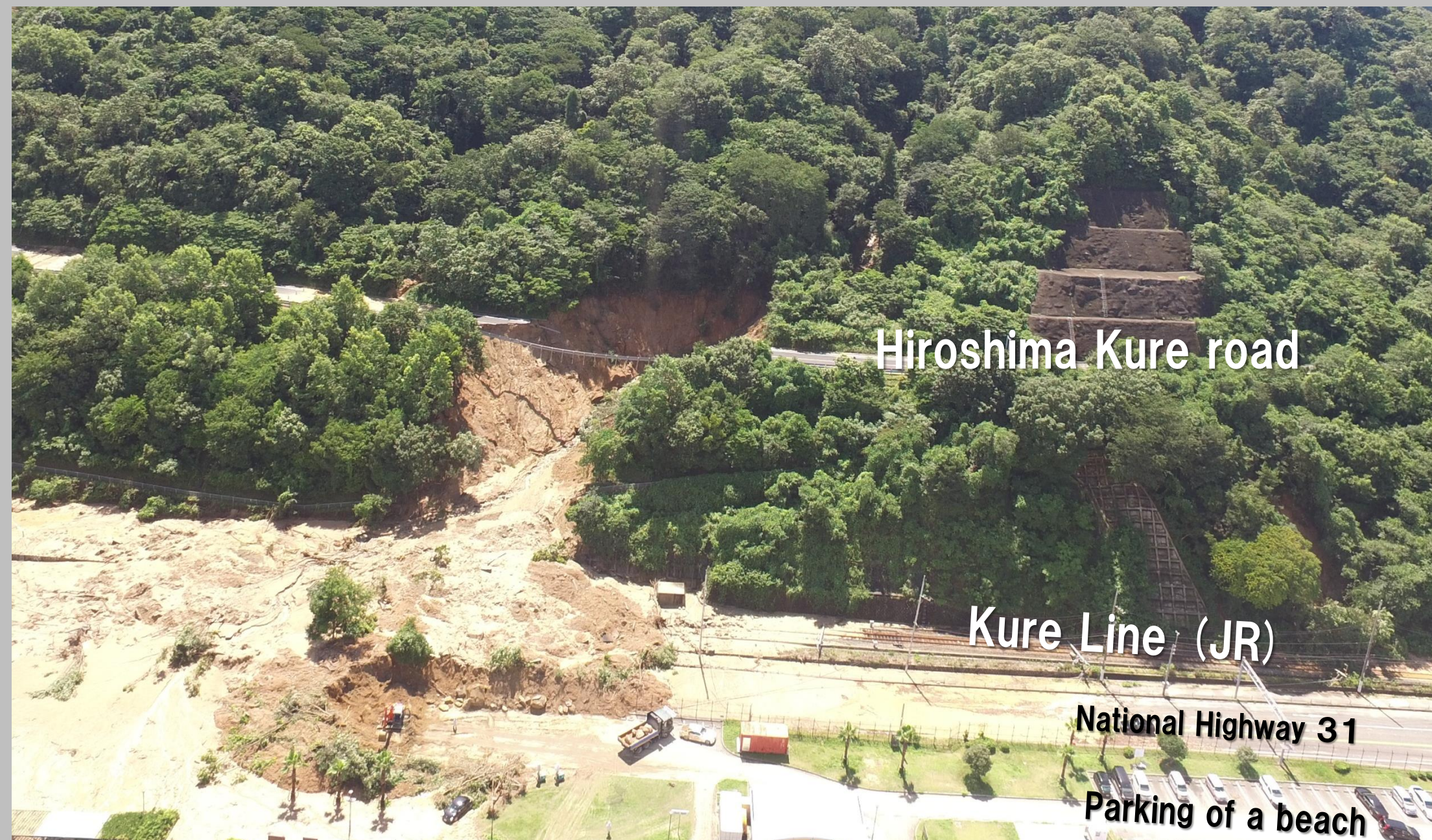
Just after the disaster (Photo: 9 July 2018)
