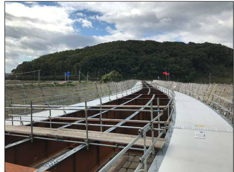
②新設橋梁
