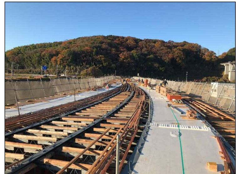
②新設橋梁
