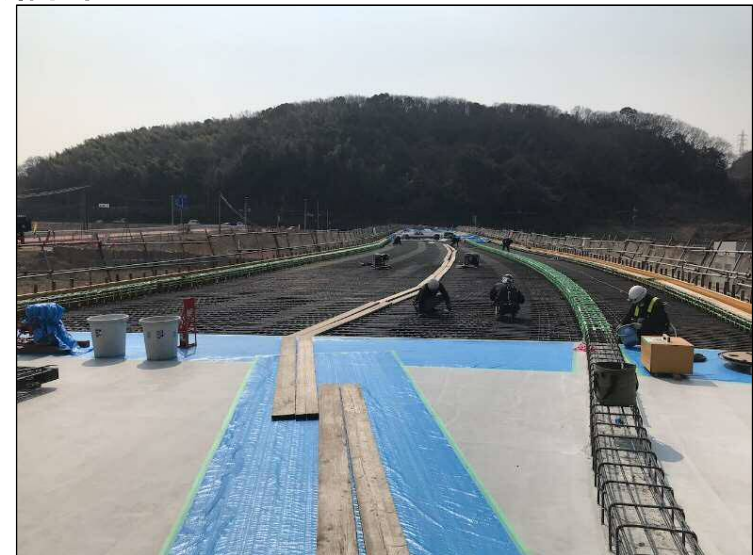
②新設橋梁
