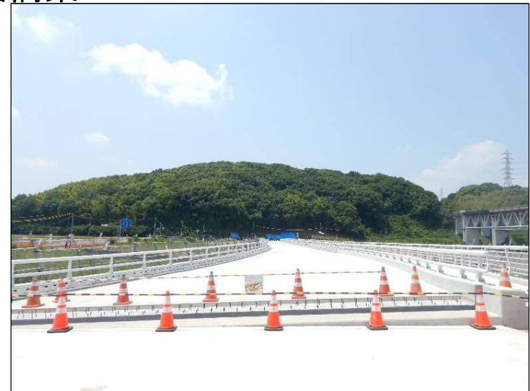
②新設橋梁
