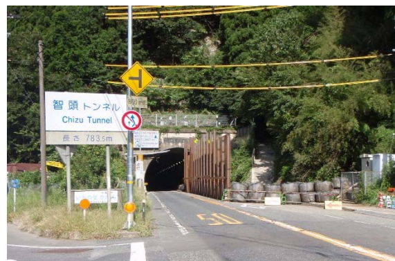
仮設防護柵(H29.6.3完)
