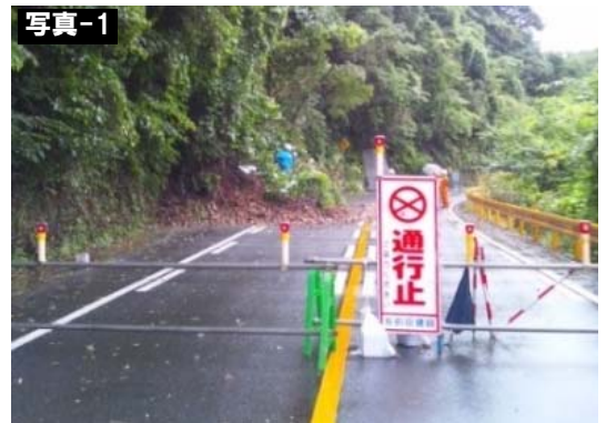
▲H25.9被災状況(長門市俵山)
